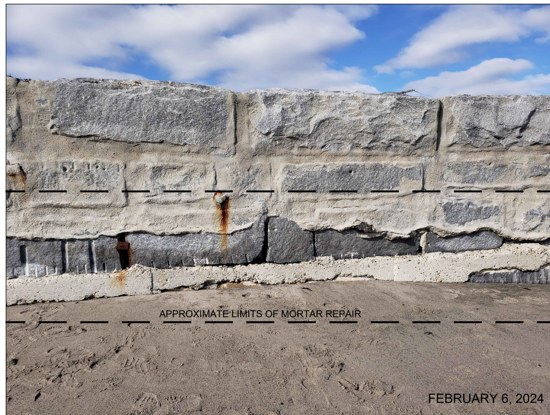
3 LOWER GRANITE BLOCK WALL REPAIR 2
