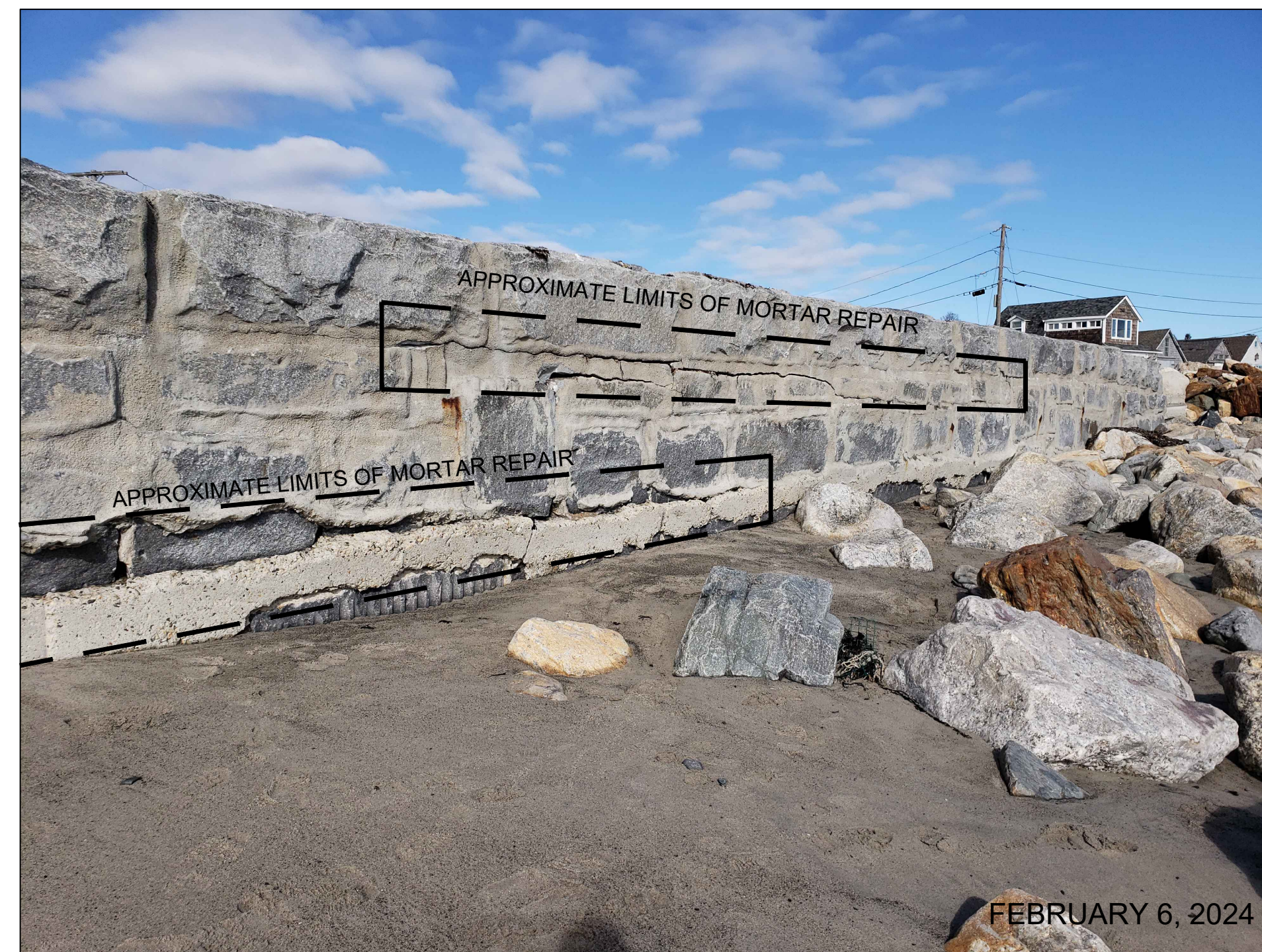
4 UPPER & LOWER GRANITE BLOCK WALL REPAIR 2
